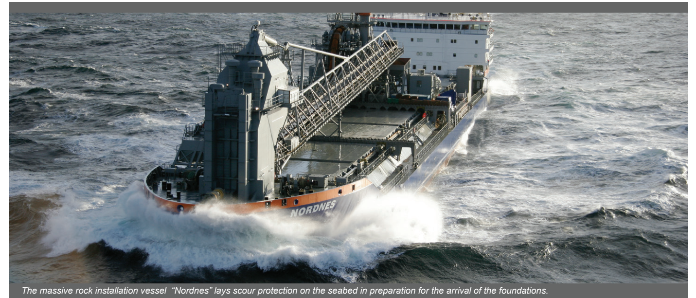
The massive rock installation vessel "Nordnes" lays scour protection on the seabed in preparation for the arrival of the foundations.
